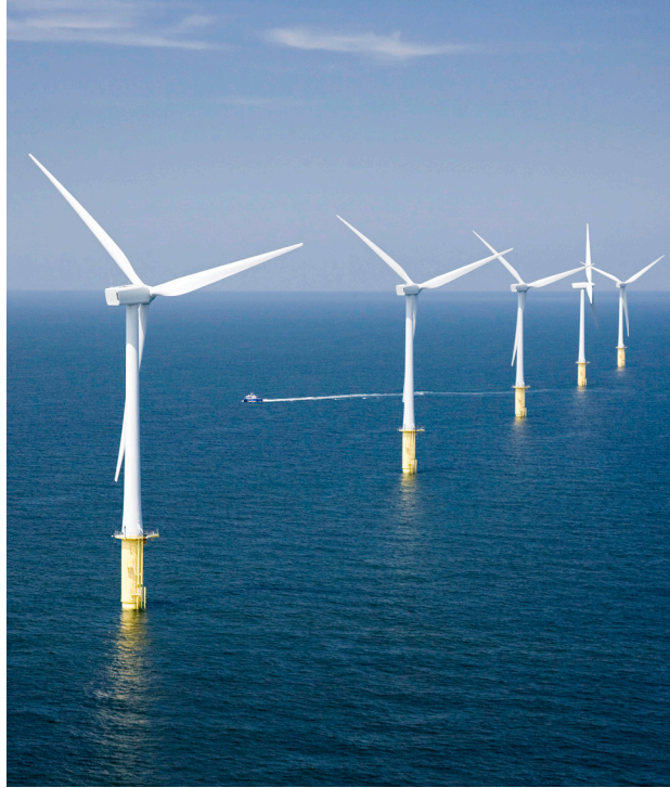
North Hoyle wind farm in Prestatyn was Wales's first offshore wind farm in the Irish Sea. © Welsh Government
